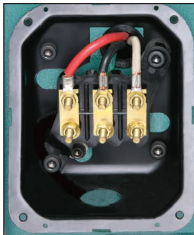
Figure 56. Power feed junction box.
