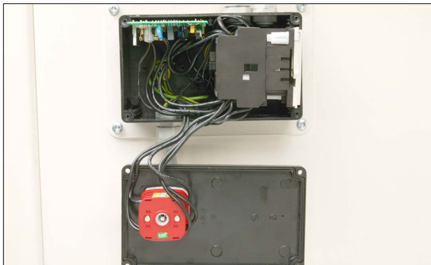
Figure 101. Main switch box wiring.
