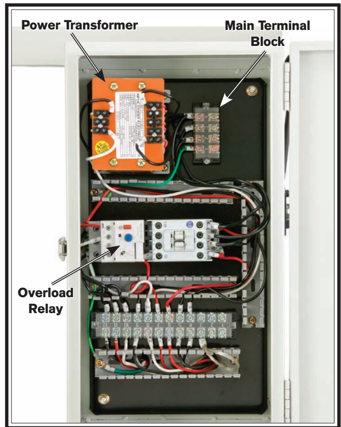
Figure 56. Electrical Box.
