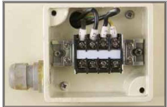
Figure 81. Lathe power-in junction box (located at right-rear of lathe stand).
