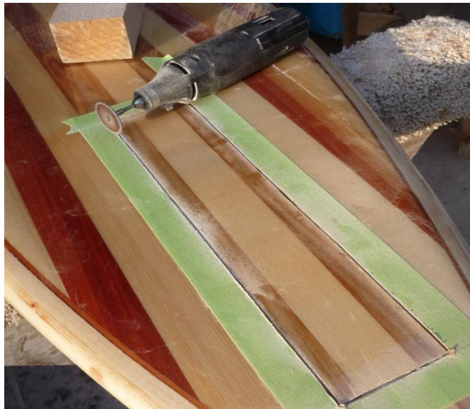
A Dremel tool and cut-off wheel are used to cut through the fiberglass and into the wood.
