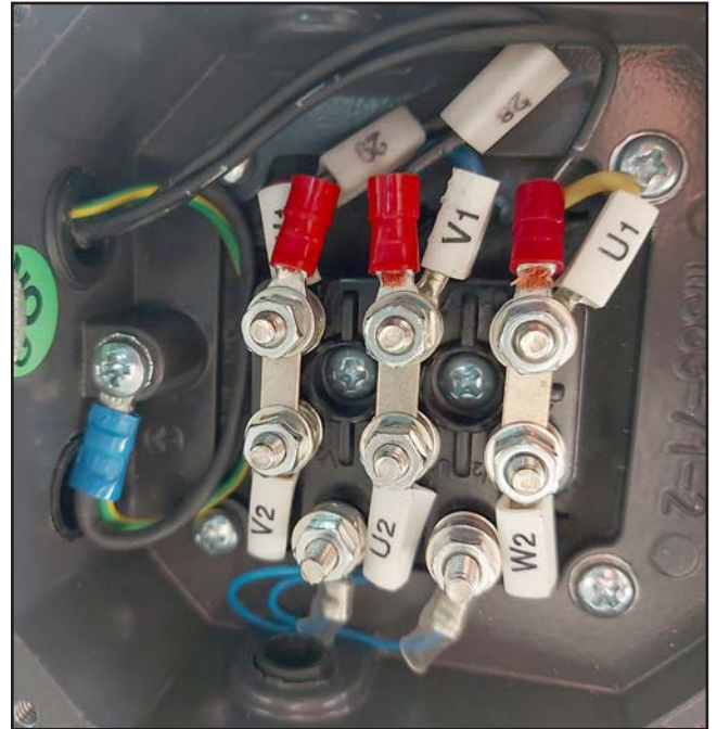
Figure 70. Oscillation motor wiring.
