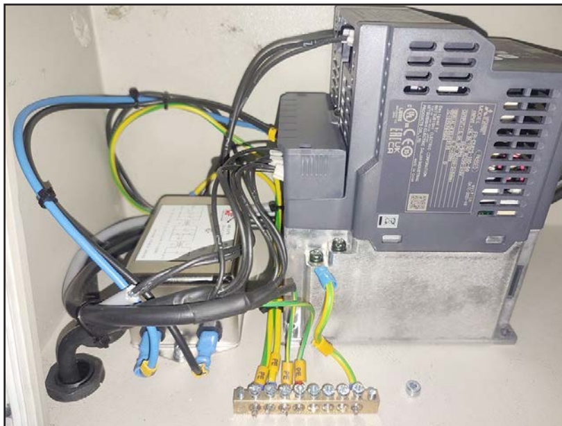
Figure 68. VFD and EMC filter wiring.
