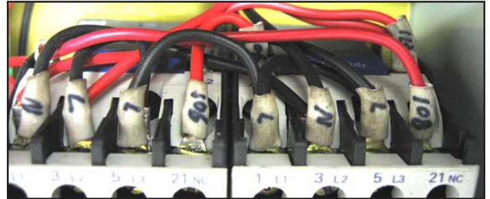
Figure 60. Contactor wiring (KM2 and KM3).
