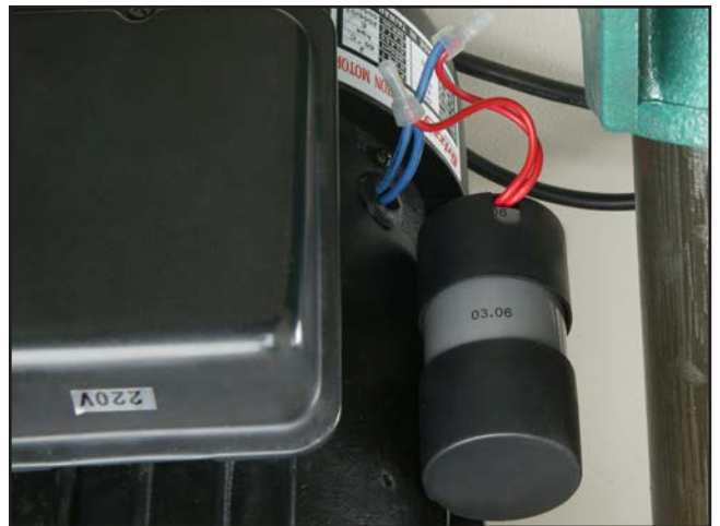
Figure 83. Run capacitor.
