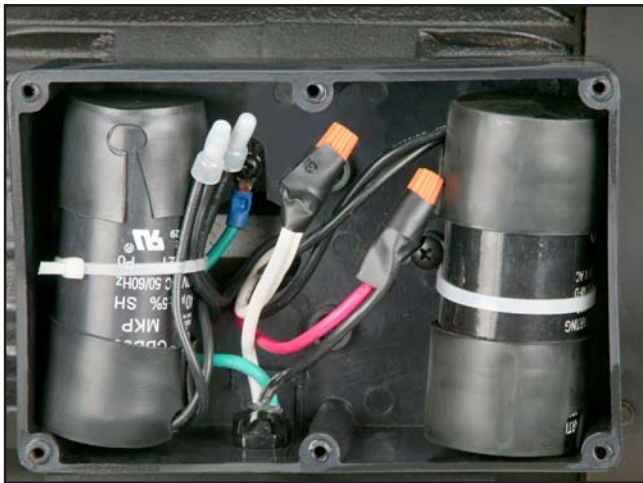
Figure 69. Motor junction box.
