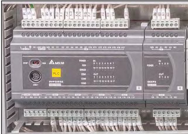
Figure 151. PLC and PLC expansion module.
