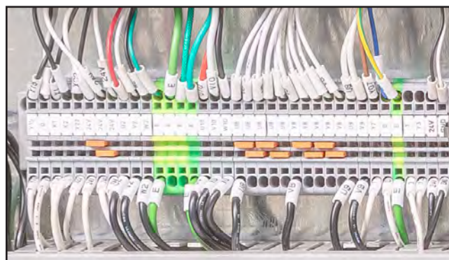
Figure 144. Terminal block (upper left).
