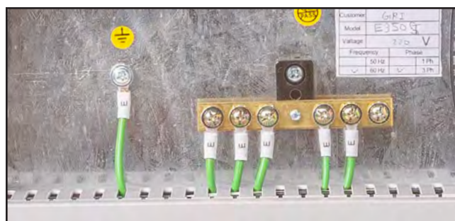
Figure 146. Grounding terminal.
