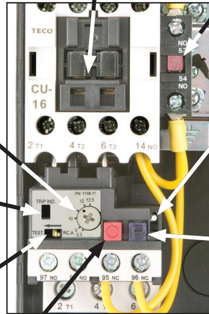
**Manual/Auto Reset Lever:** In the up position, the thermal relay is in manual reset mode. This means you must re-install the outside cover and push the red OFF button, then push the green ON button to reset the thermal relay. In the down position, the thermal relay will automatically reset when it has cooled.
