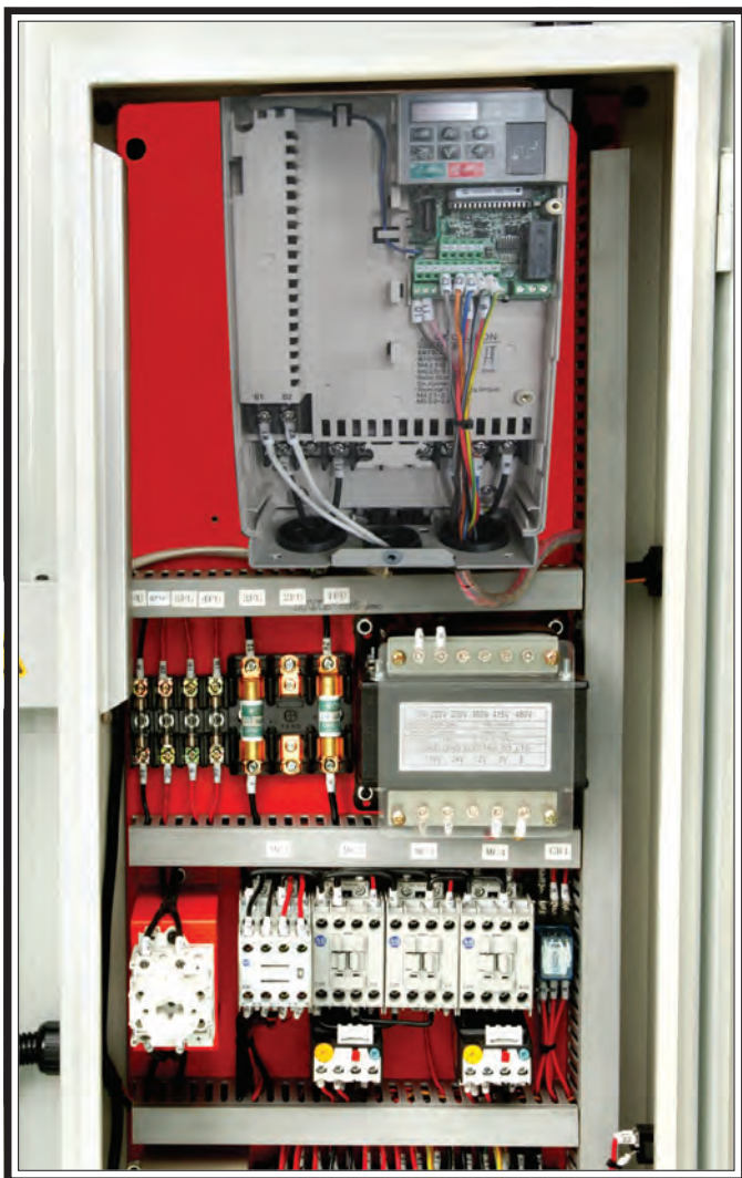
Figure 69. Electrical cabinet wiring.
