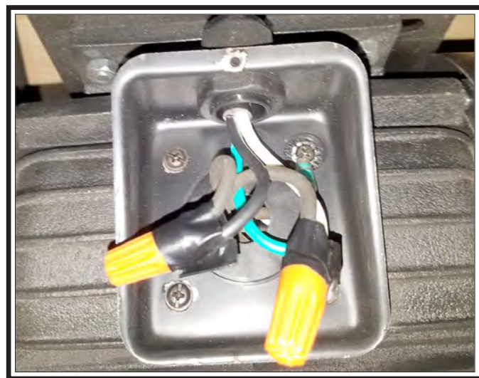
Figure 59. Main motor junction box.
