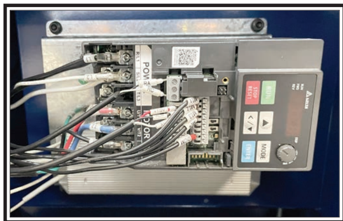
Figure 60. VFD wiring.
