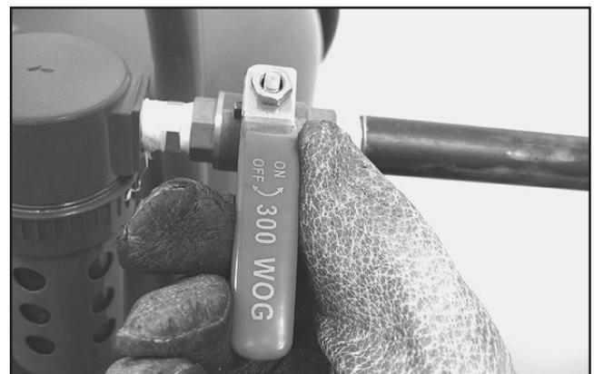
**Figure 8.** Tank air supply valve, closed.
