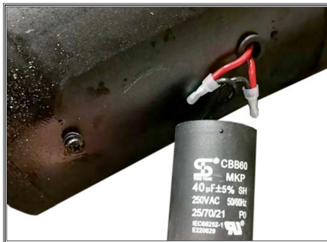
Figure 11. Run capacitor.
